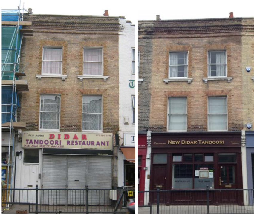
Figure 2: 347 Caledonian Road before and after shopfront restoration
